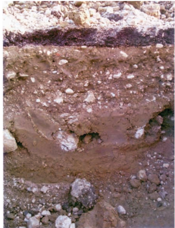
Fig. 8 Soil layer of asphalted road
