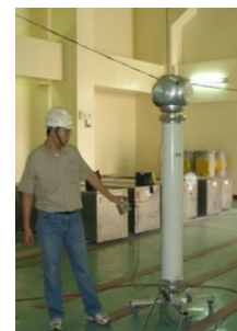
(a) Coupling capacitor
